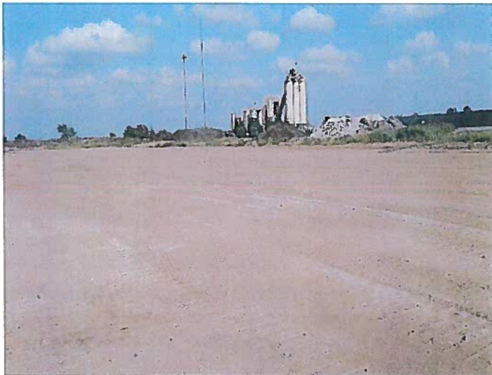
GRAVEL REMOVED, SITE GRADED TO PRE DEVELOPMENT ELEVATIONS, TOPSOIL PLACED
