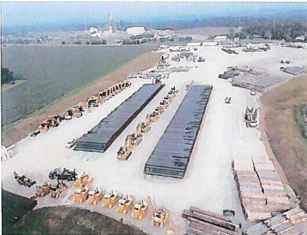
CONTRACTOR YARD PRIOR TO PIPELINE CONSTRUCTION
