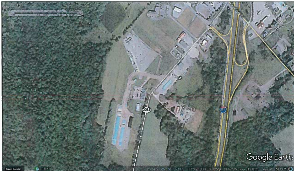
CONTRACTOR YARD DURING PIPELINE CONSTRUCTION DTE BLUESTONE PIPELINE NEW MILFORD, PA
