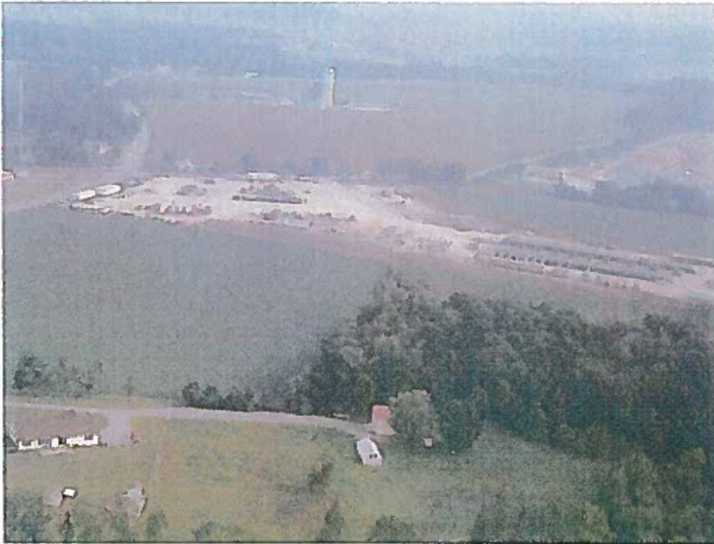
CONTRACTOR YARD PRIOR TO PIPELINE CONSTRUCTION
