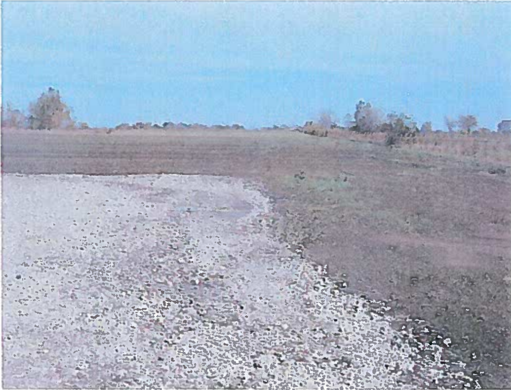
BEGIN CONTRACTOR YARD CONSTRUCTION – GRAVEL PLACEMENT
