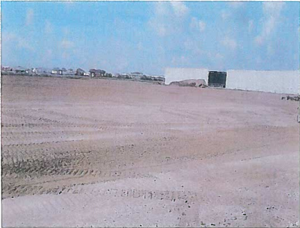
GRAVEL REMOVED, SITE GRADED TO PRE DEVELOPMENT ELEVATIONS, TOPSOIL PLACED
