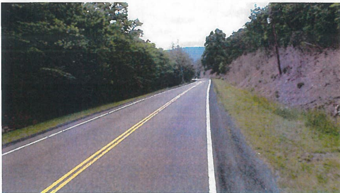
Route 42 along property frontage (west of Route 254)
