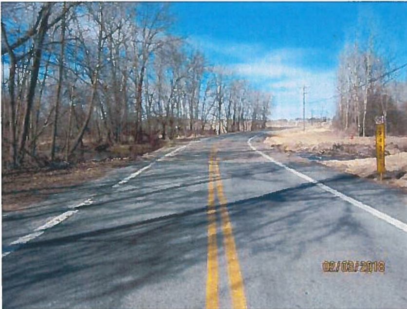
South approach. Note curve at the north approach and the water height gauge.
