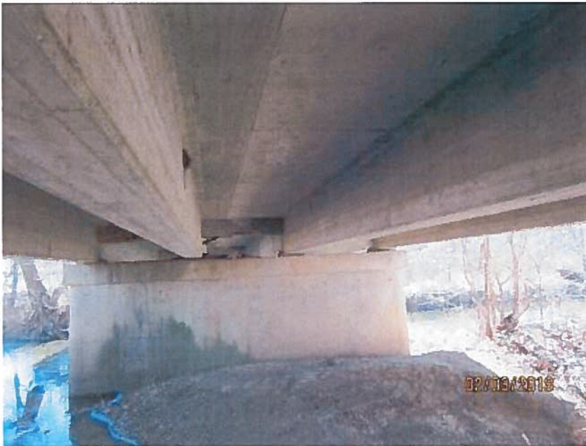
General condition of superstructure. This is Span 3.
