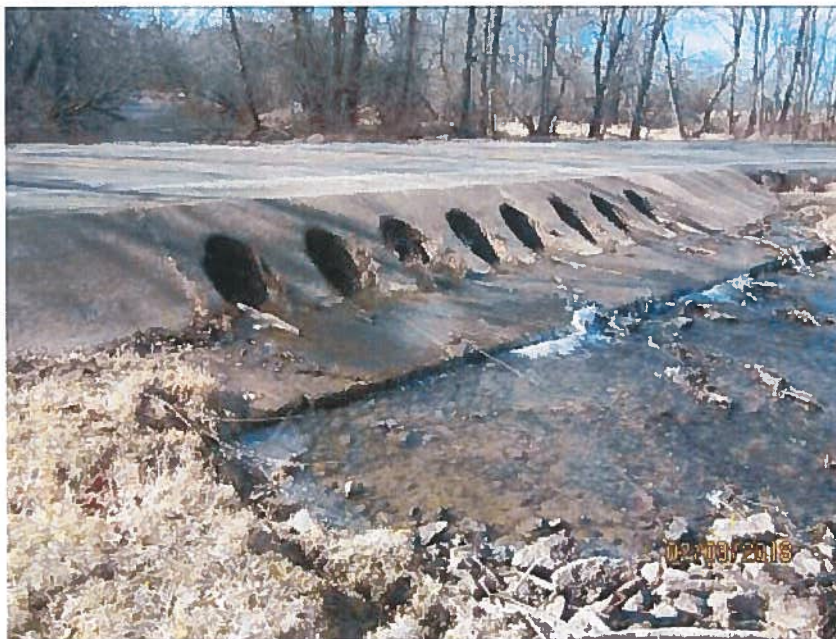
General condition of pipe outlets and endwall.
