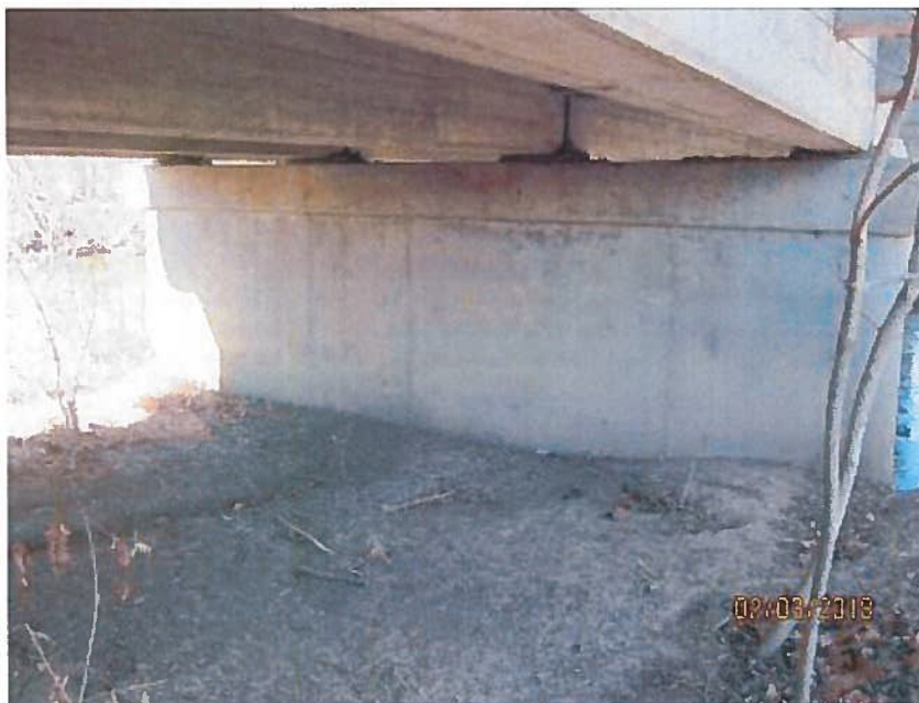
General condition of Piers. This is Pier 1.
