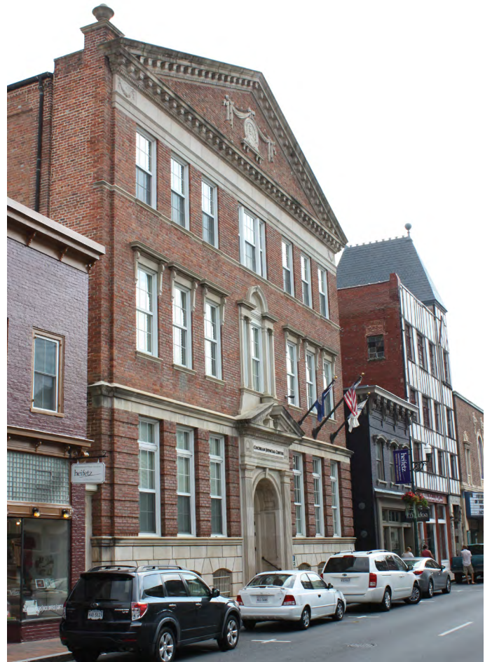
The Cochran Judicial Center with its 1929 redesigned facade by Sam Collins retains its classical design. A side garden and walk lead to a handicapped entrance. (not shown)
