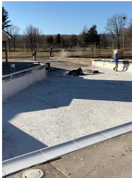
Construction progress December 2019
