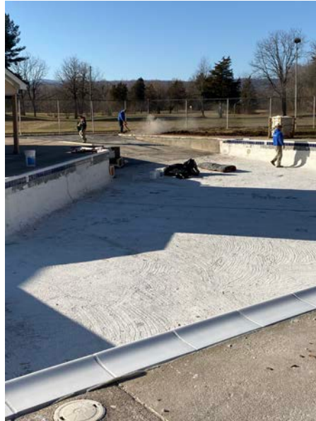
Construction progress December 2019
