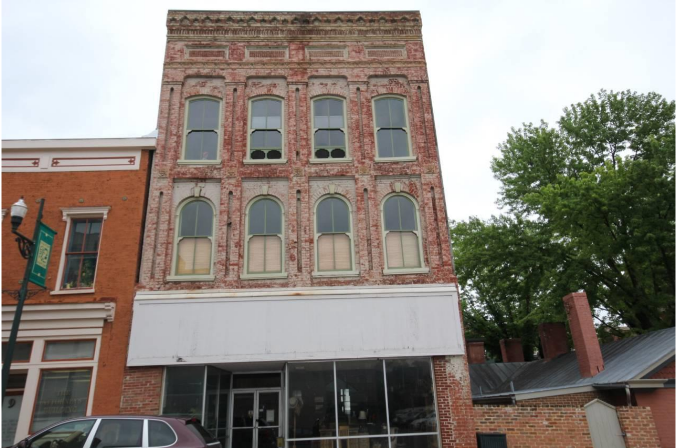
11 South Augusta Street
