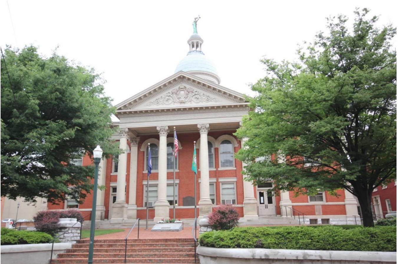
1 East Johnson Street
