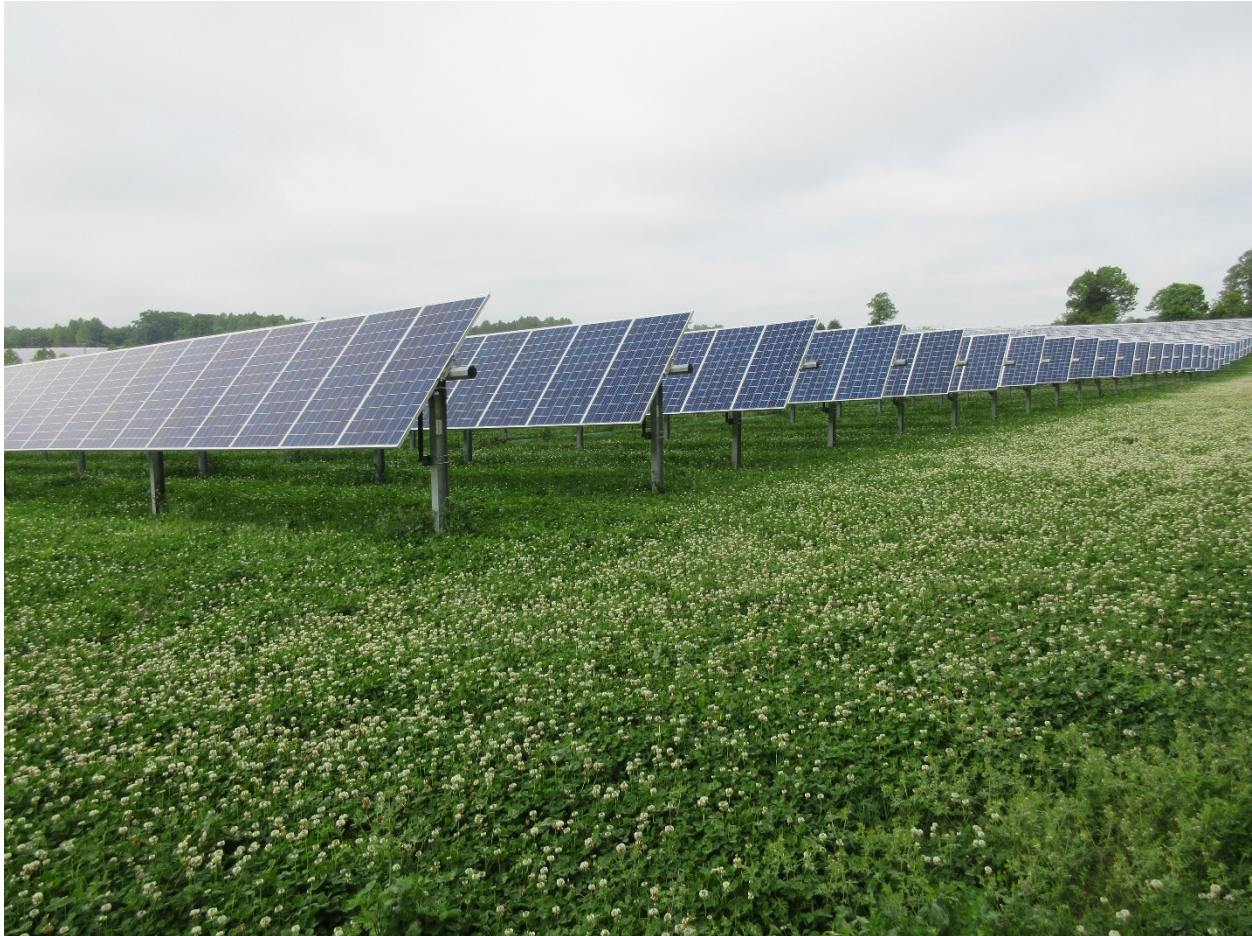
Figure 2 – Typical Single-Axis Tracker System
